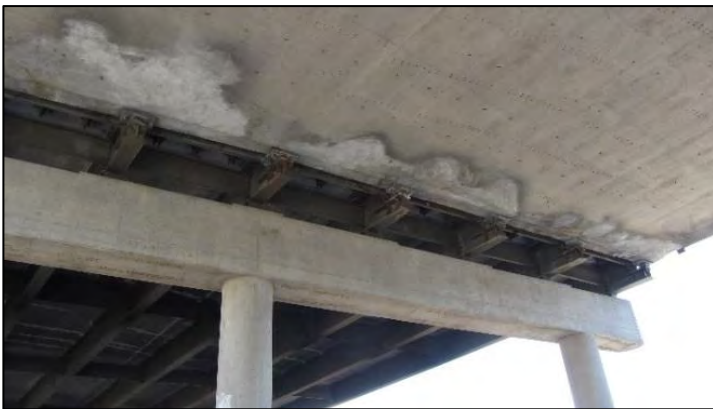
Figure 167. Unsound patched areas and efflorescence on underside of RC voided slab for Bridge Number 15558X.
