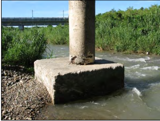
Figure 153. Exposed column footing in stream.
