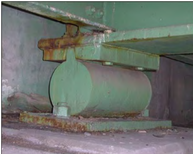
Figure 146. Surface rust on moveable bearing.
