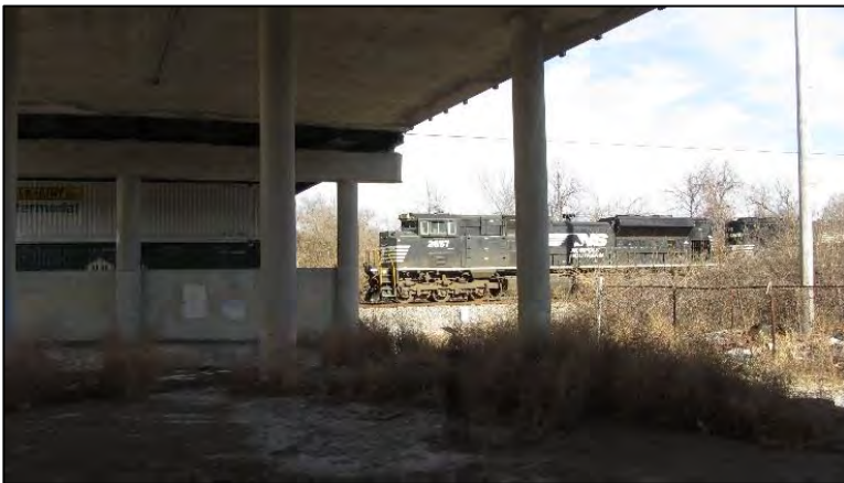
Figure 114. Freight train passing below Bridge Number 15558X
