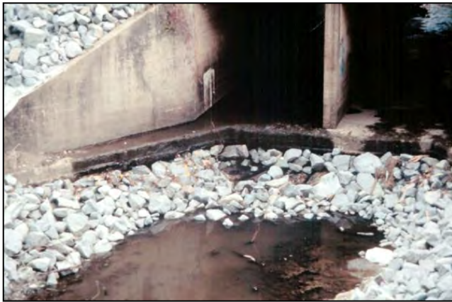
Figure 152. Scour and missing riprap at concrete box culvert outlet.
