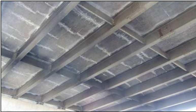
Figure 161. Transverse cracking with efflorescence on underside of RC deck for Bridge Number 15558X.
