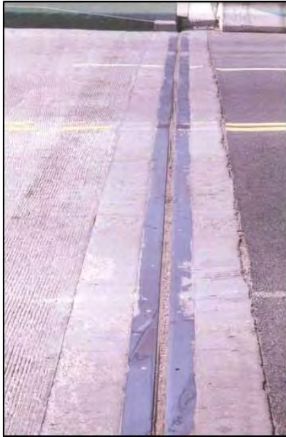
Figure 147. Joint partially filled with debris.
