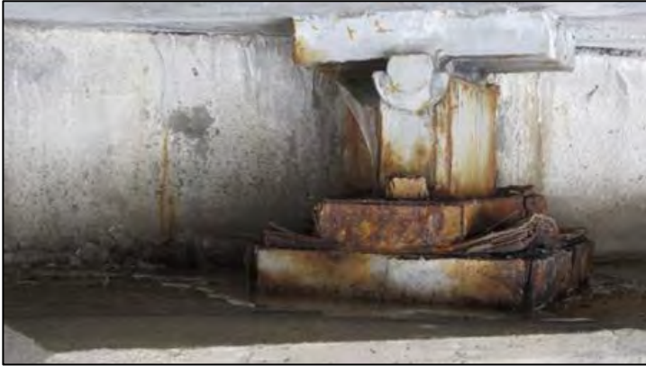
Figure 173. Typical rocker bearing with movement restricted by pack rust for Bridge Number 15558X.
