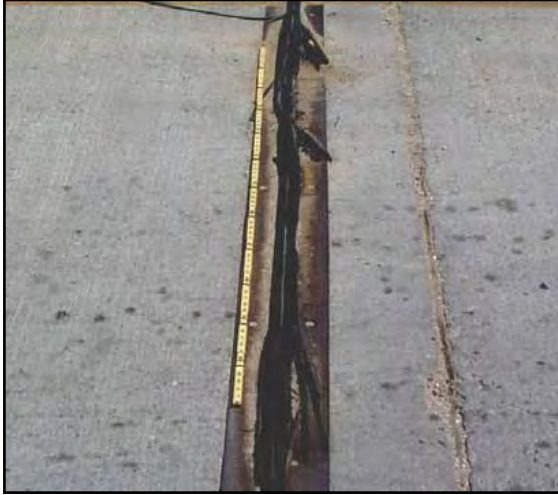
Figure 149. Joint seal is torn and partially pulled out.
