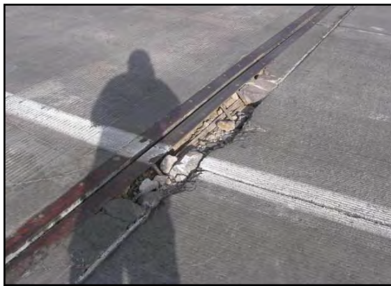
Figure 148. Spill in joint header. (Source: Colorado DOT)
