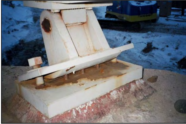
Figure 145. Misaligned rocker bearing. (Source: Alaska DOT)
